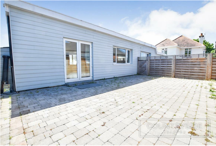
Shed 18'3" x 7'6" (5.56m x 2.29m) Power and lighting
